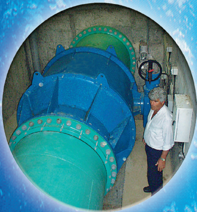
DIGA DI ARMINOU (CYPRUS) NEEDLE VALVE ND 1400 ELECTRICALLY OPERATED
